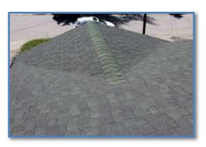
The northern facing slope is showing some moss growth. While moss itself does not damage the roof surface, it does retain water, making it harder for the roof to dry out between precipitations. A wet roof tends to age more
