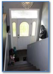
• The stairway from entry level to main floor is missing a hand rail. Install for safety and convenience.
