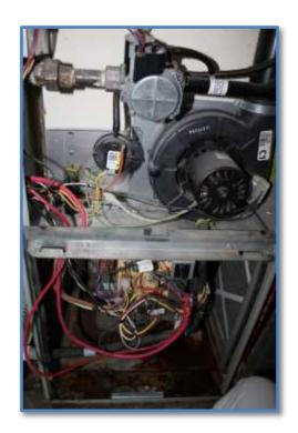
Heating systems last longer and perform more efficiently when serviced every other year. This furnace, while fully operational, is in need of servicing.
