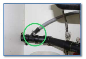
• The dishwasher does not have a high loop installed in the drain line. A high loop is meant to prevent wastewater from being siphoned back into the dishwasher and contaminating its contents. Install high-pool as needed.
