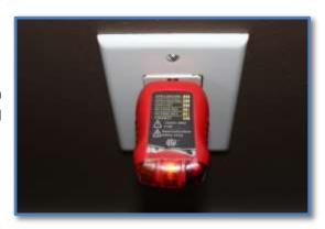
• The GFCI-rated outlet in the main floor bathroom does not reset and outlet may be faulty. Assess and correct as needed.
