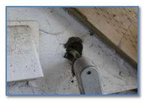
• A loose electrical conduit body was found under the balcony stairs. Re-anchor to wall as needed.
