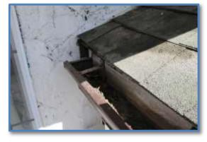
• Monitor gutter at the roof over the front porch as is slopes towards the home and may spill / splash onto the stucco if the gutter and nearby downspout are plugged (they are currently plugged).
