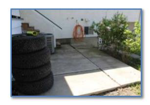
Movement and differential settling has occurred between the various concrete slabs. Movement may continue or may have slowed down. Monitor and maintain as needed. Watch for trip hazards.
