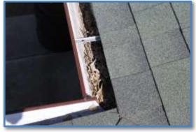
• Monitor gutter at the roof over the front porch as is slopes towards the home and may spill / splash onto the stucco if the gutter and nearby downspout are plugged (they are currently plugged).
