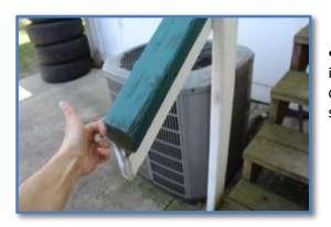
• The hand rail to the sun deck is wobbly and lacks integrity. Replace hand rail with spindled hand rail for safety and convenience and to protect children from falling off the stairs sideways.
