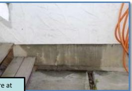
Substantial amount of moisture at the exterior wall and foundation
