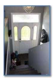
• The stairway from entry level to main floor is missing a hand rail. Install for safety and convenience.
