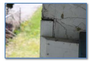
• Keep all exposed wood surfaces, including facia, soffits, gable ends, well-painted to protect against weathering and deterioration.
