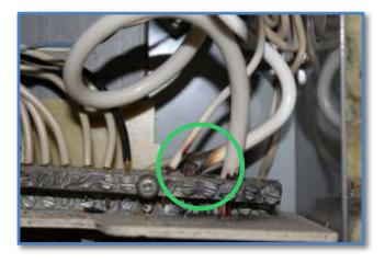
• A transformer was found inside the main electrical panel. This is poor practice. Transformers should be installed outside the electrical panel as per electrical regulations. Correct as needed by a licensed electrician.
