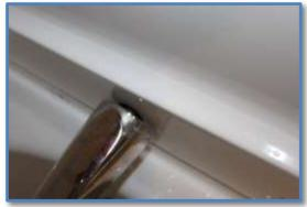
• Silicone caulking is needed in various locations within and along the tub / floor to help protect vulnerable areas against water penetration. It is probably easiest to remove all old and stained caulking and to start again instead of attempting to touch-up.
