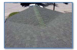
The northern facing slope is showing some moss growth. While moss itself does not damage the roof surface, it does retain water, making it harder for the roof to dry out between precipitations. A wet roof tends to age more
