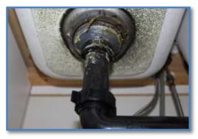
• While no leak was observed, caulking and connections under the left-hand sink look troublesome. Monitor until ensured there are no latent leaks.
