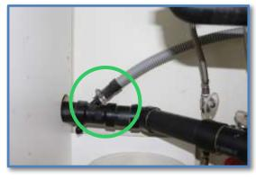
• The dishwasher does not have a high loop installed in the drain line. A high loop is meant to prevent wastewater from being siphoned back into the dishwasher and contaminating its contents. Install high-pool as needed.
