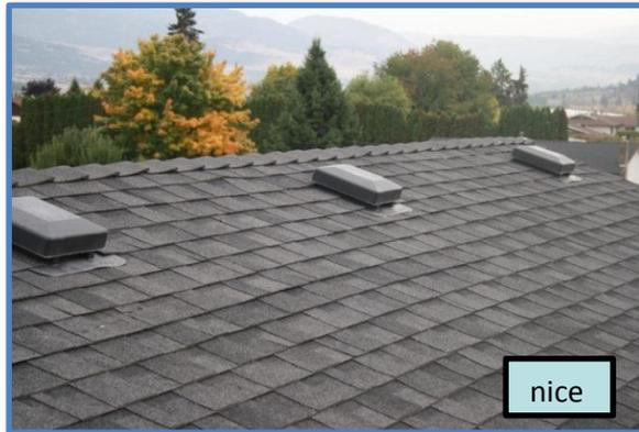
Roof penetrations (plumbing stack, roof vents, etc) seem to be in satisfactory condition from what could be seen. Roof penetrations should be checked for cracks and breaks, proper caulking as part of regular roof maintenance. Exposed nails should be sealed.
