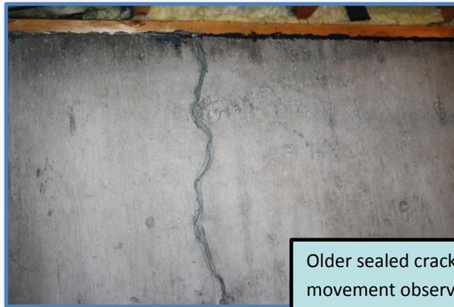
Older sealed crack, no new movement observed.
