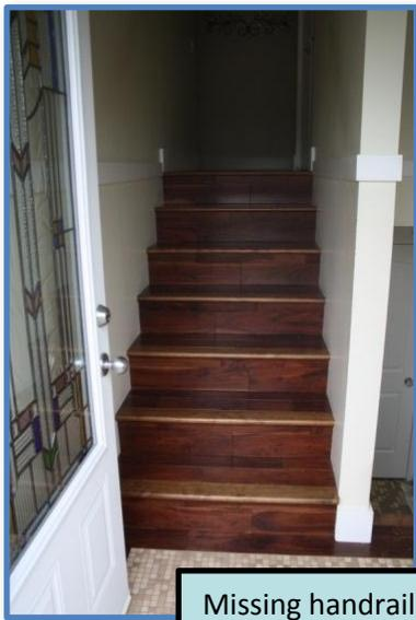
The interior staircase leading to the main floor, as well as the staircase leading to the basement, does not have a hand rail. While acceptable for the era of the home, it is recommended for safety reasons that stairs with more than three risers to have hand railings installed.
